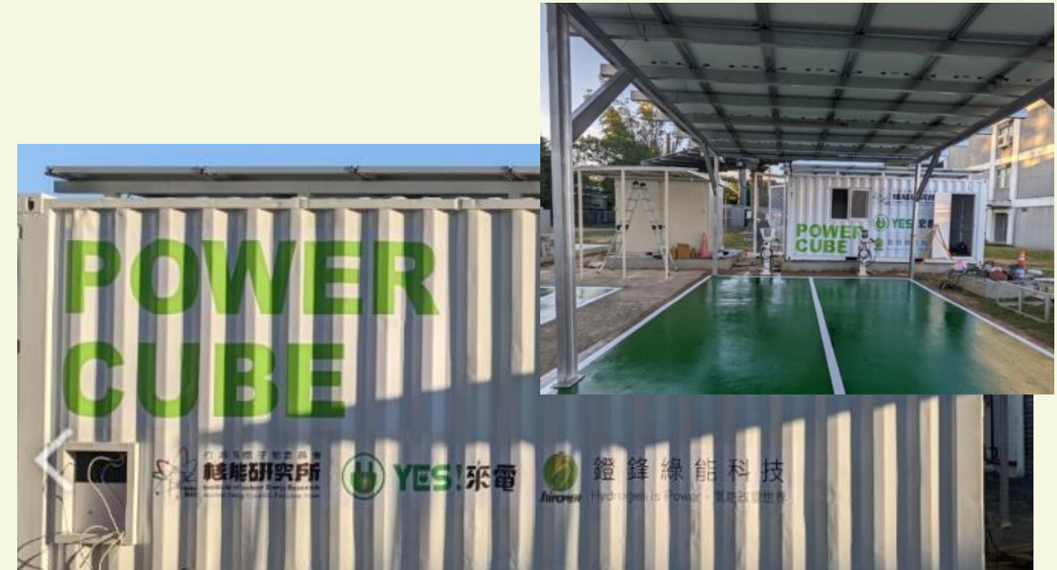
10kW PV + 60 kWh energy storage + EV charger (micro grid and energy storage)
